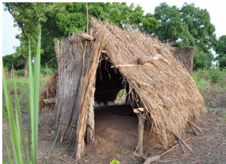
Household latrine constructed by community members with locally available materials.
