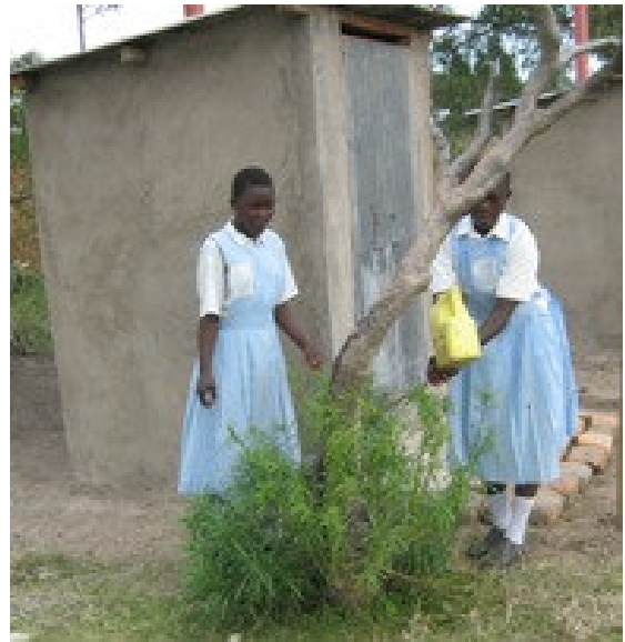
Latrine built with the improved technology with the pupils using the tins to wash their hands after a visit to the latrines.
