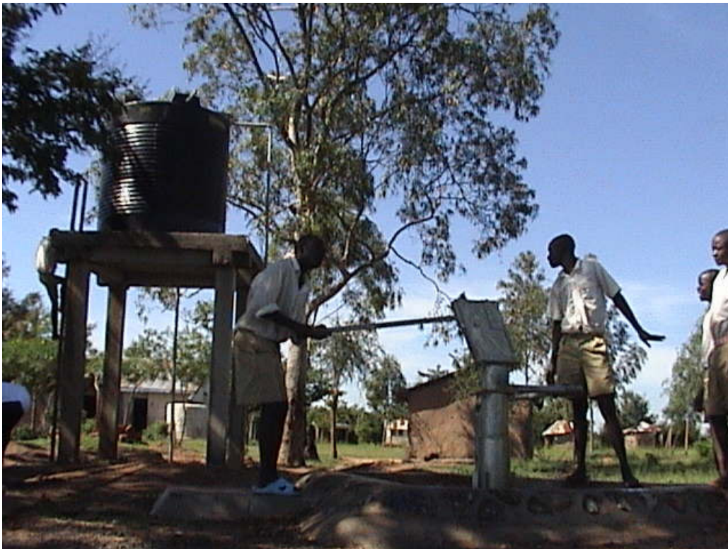
Students at Mbeme primary school as they pump water into storage tank serving the school and community.
