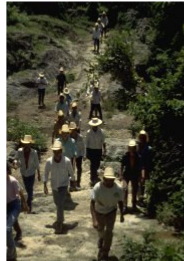
Community members walk along path of conduction line which is buried in concrete and rock beneath path. El Limón.
