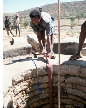
Well construction in Wersege, Tigray.
