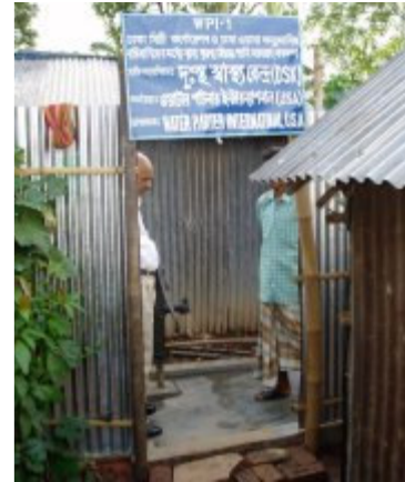
A new Pallabi Slum water point constructed under the WPI project.
