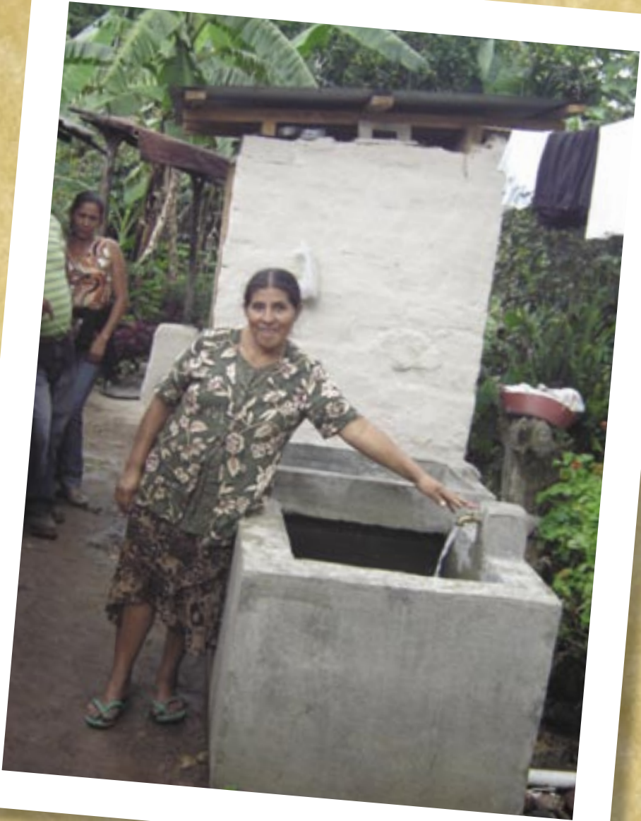
Clementina stands by her family's new water connection with a cement basin for washing. These basic utilities have transformed her day-to-day life.
